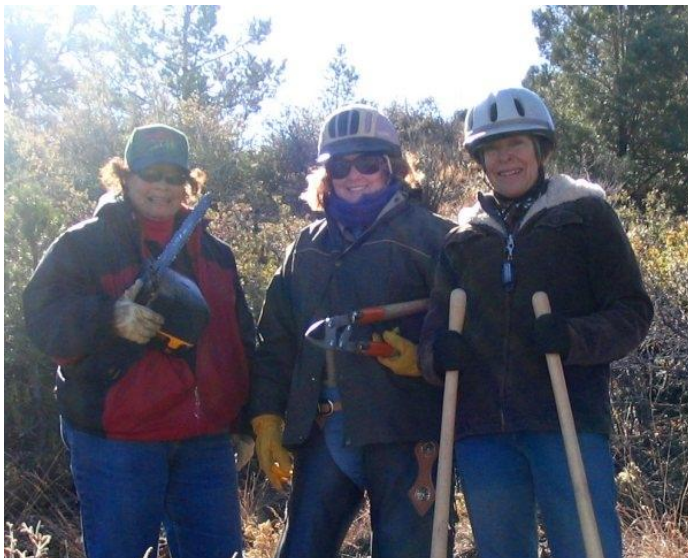
Clearing crew on just finished Almosta Trail
